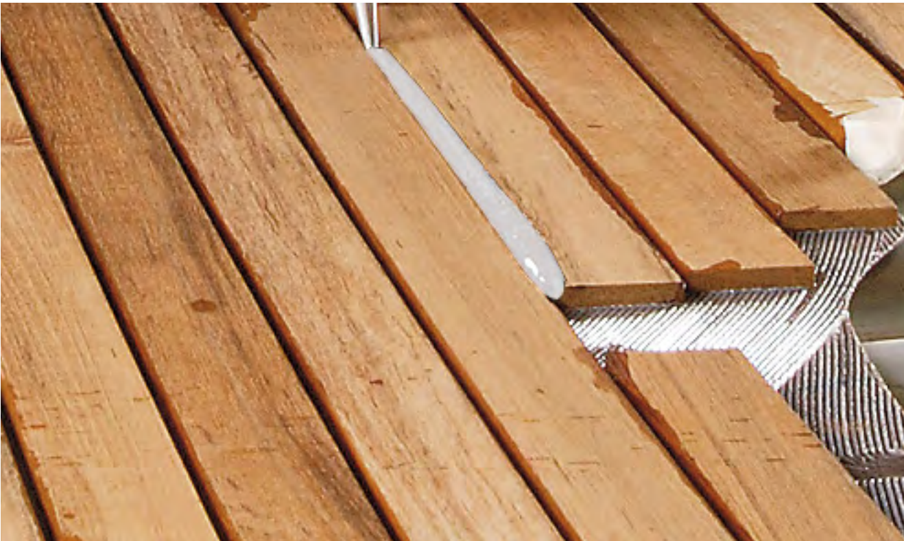
With dispersion adhesives, for example, ship decks made of wood are glued. In this case, the water resistance of the adhesive is required.
