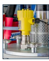
Radar sensors for level control
